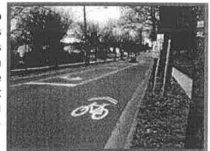
Shared Lane Marking
