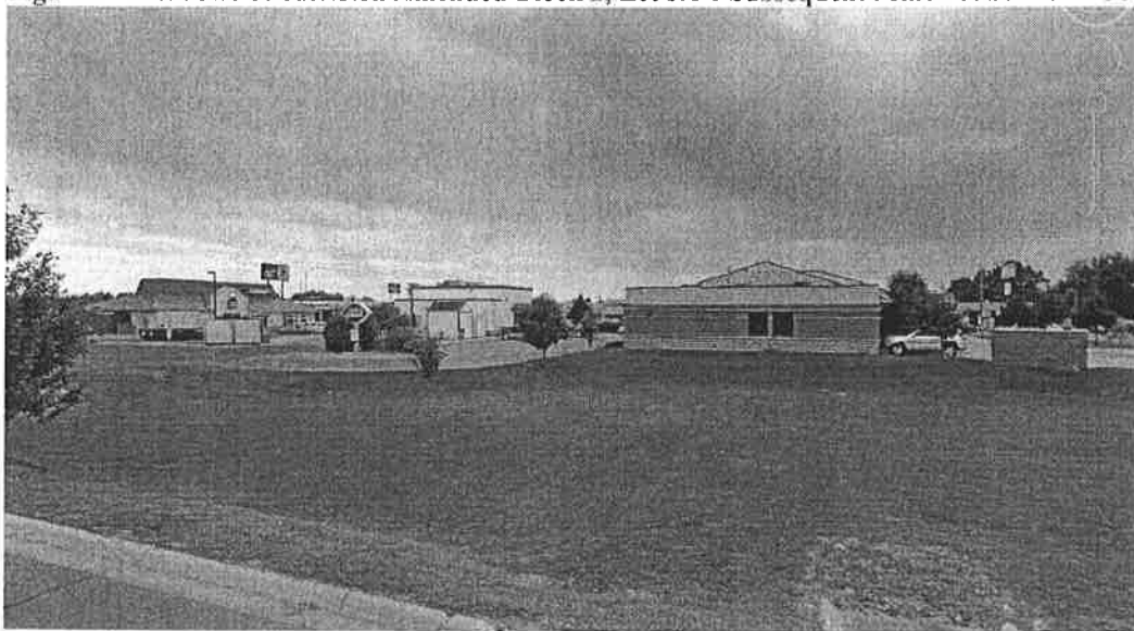
Figure 3: Meadows Subdivision Amended Block 2, Lot 3A-1 Subsequent Minor Subdivision Property Image
