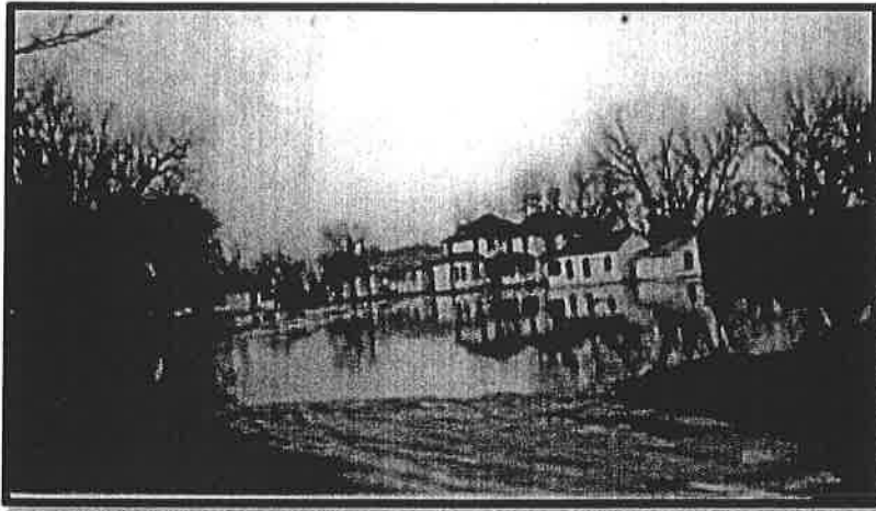
Figure 5: Pleasant Street Flooding 1944 (Montana's Flooded Past, 2011)
