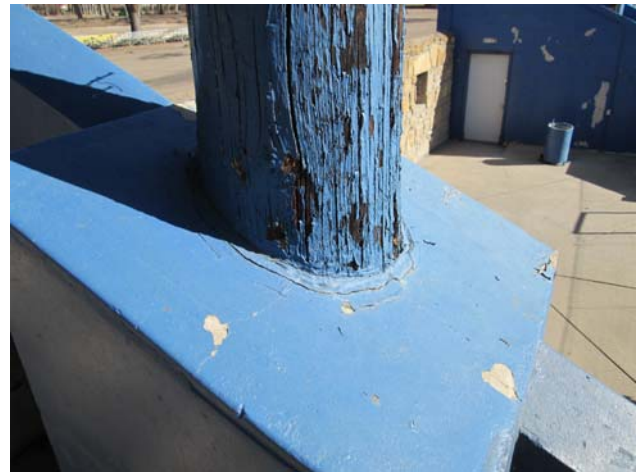
Photo 6 – Wood Pole Base
