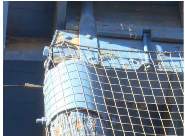
Photo 4 – End Condition of Beam Assembly
