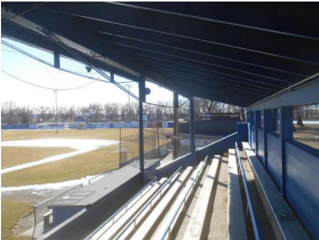
Photo 3 – Stadium Tension-Rod Beam Assemblies
