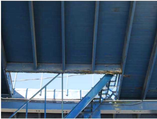
Photo 1 – Stair Opening in Roof
